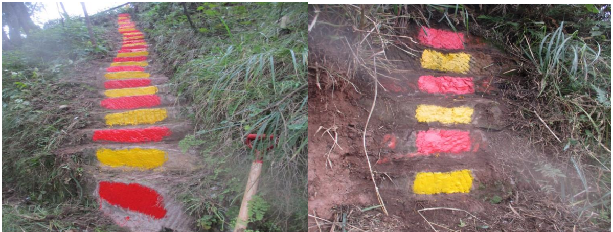
管道作业带沿线浆砌石挡墙堡坎
